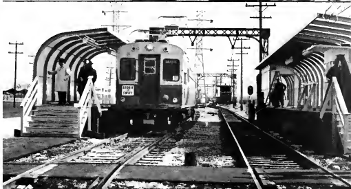
By April 10, training trips were being made to qualify men for train operation, and platform construction was nearing completion at Dempster. The arriving platform is at left; the southbound platform, at right.
